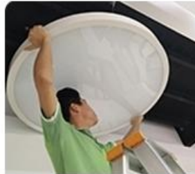
1. Install the ceiling parts in the wall.
